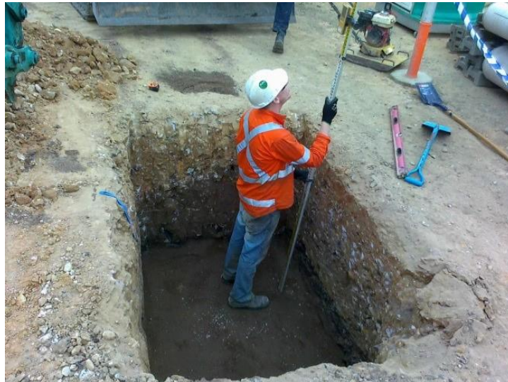
Checking the base
