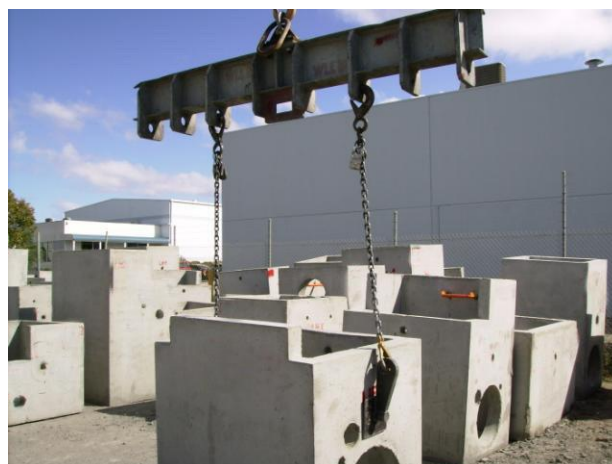
Lifting with spreader bar
