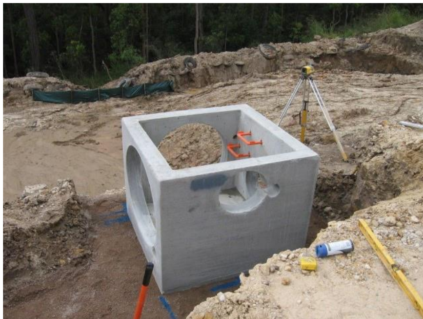
Pit positioned on leveled bedding material
