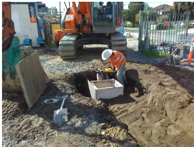
Compaction of backfill around pit
